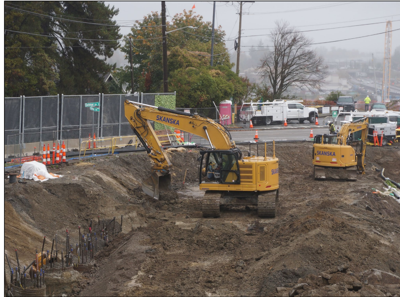
Crews excavating at lid pier 4 near Roanoke Park (September 2026)
