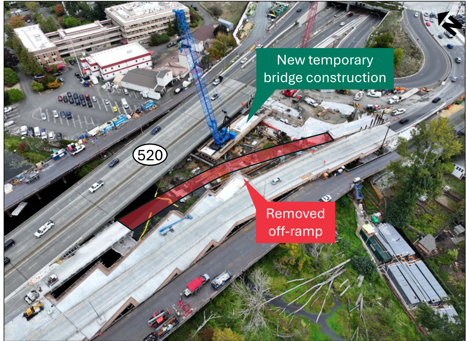
Progress on removing the old off-ramp and the new bridge (September 2026)
