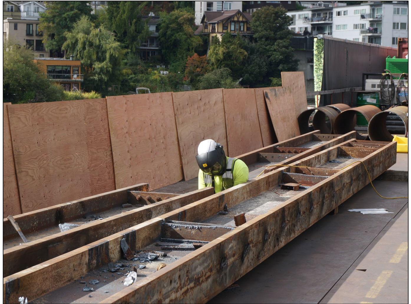
A welder assembling steel framing on the temporary work trestle (October 2026)
