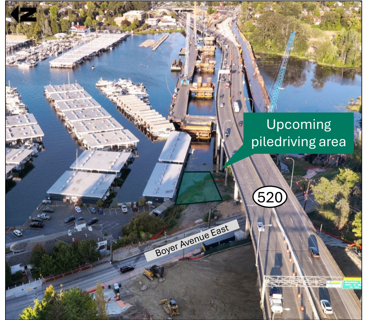
Graphic showing the piledriving area on the northwest corner of the work trestle.
