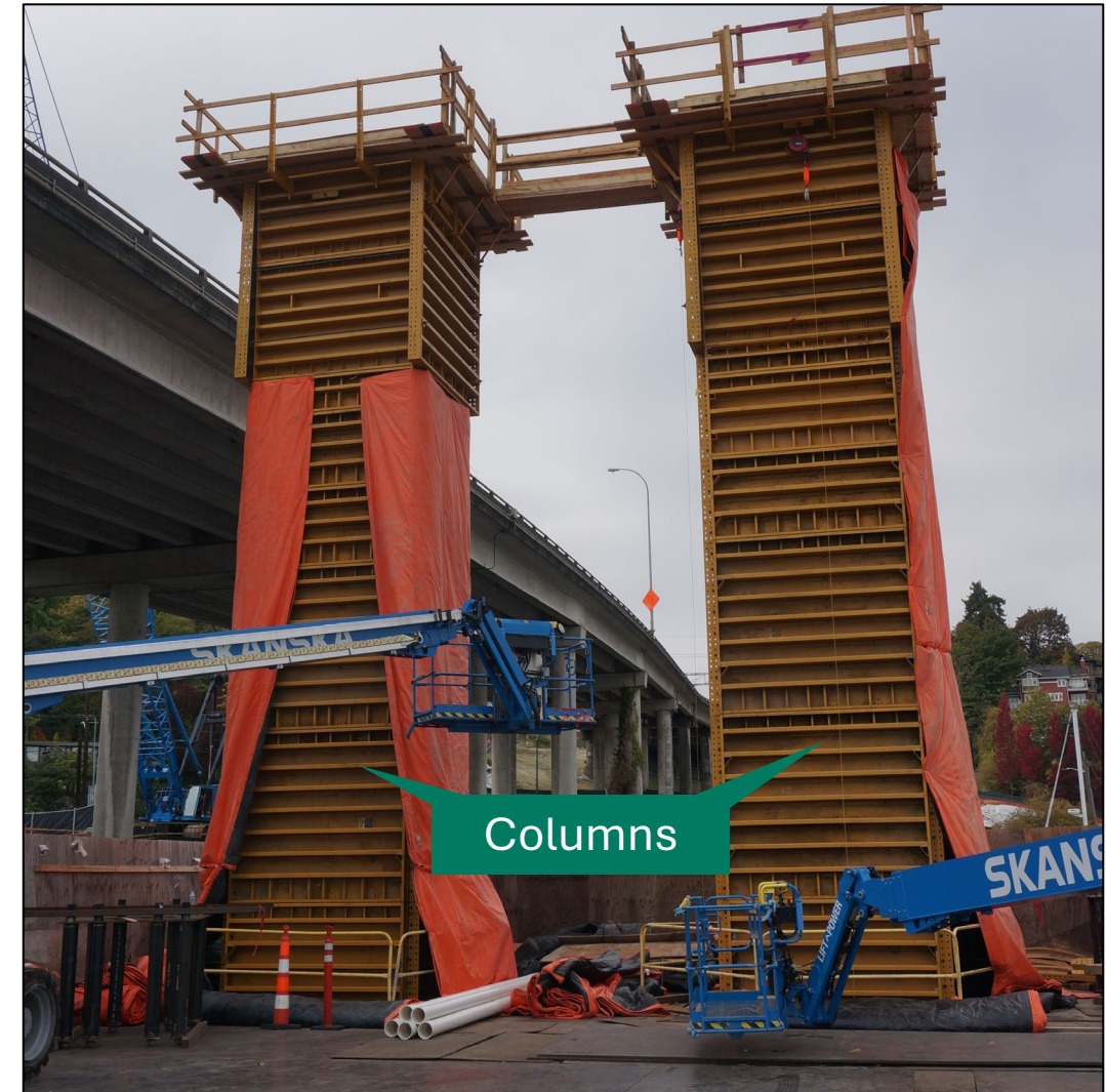
Bridge pier 4 column formwork (October 2026)
