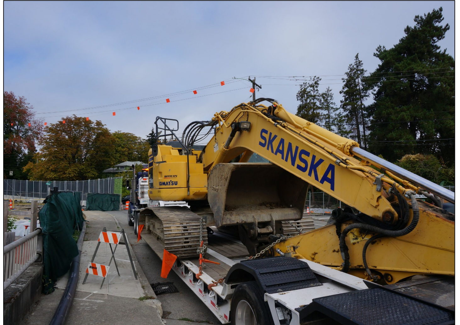
Crews transporting an excavator to the work area near Roanoke Park (October 2026)
