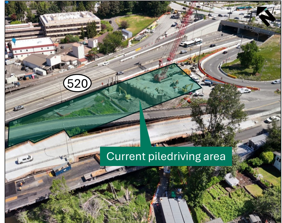
Piledriving area between SR 520 and the eastbound SR 520 off-ramp to Montlake Boulevard.
