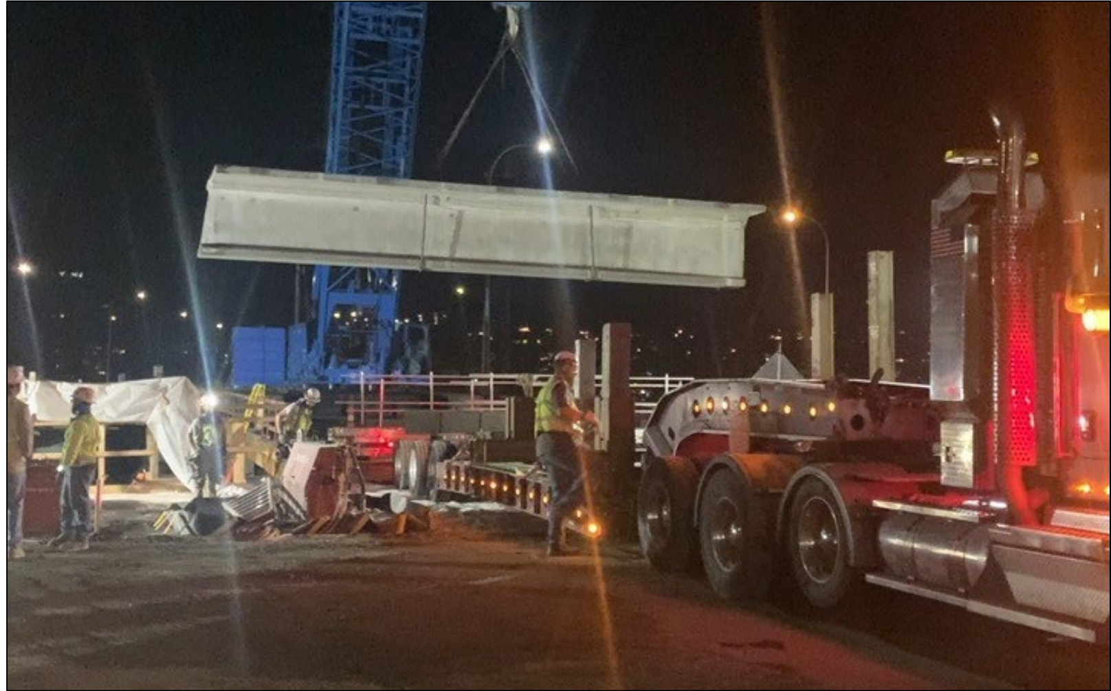
Crews using a crane to remove a section of the old off-ramp (October 2026)
