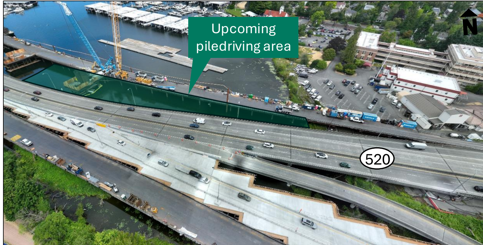
Piledriving area along the work trestle near the Montlake lid.
