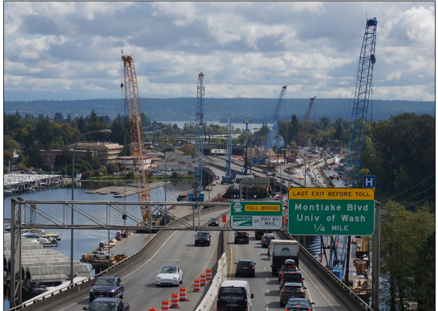
SR 520 and cranes on the work trestles looking east (September 2026)
