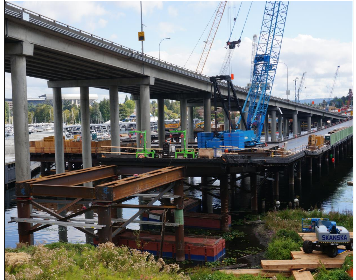
The southwest corner of the work trestle looking east (September 2026)
