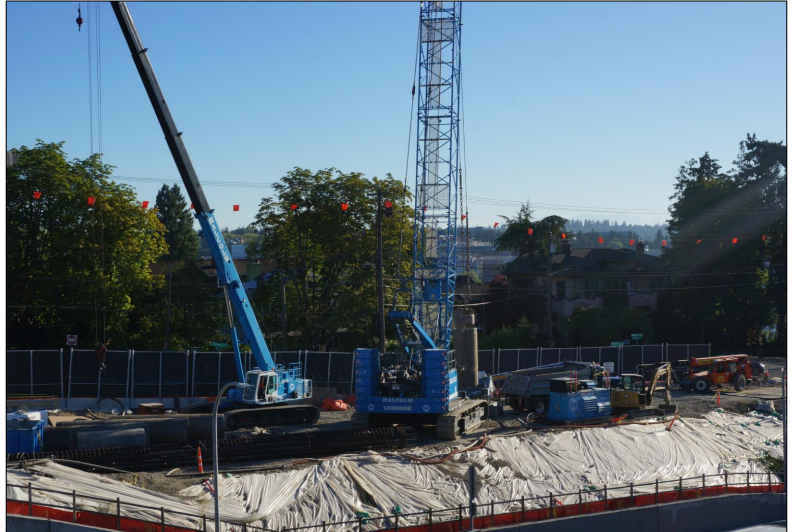
Crews installing lid pier 4 near Roanoke Park (July 2026)
