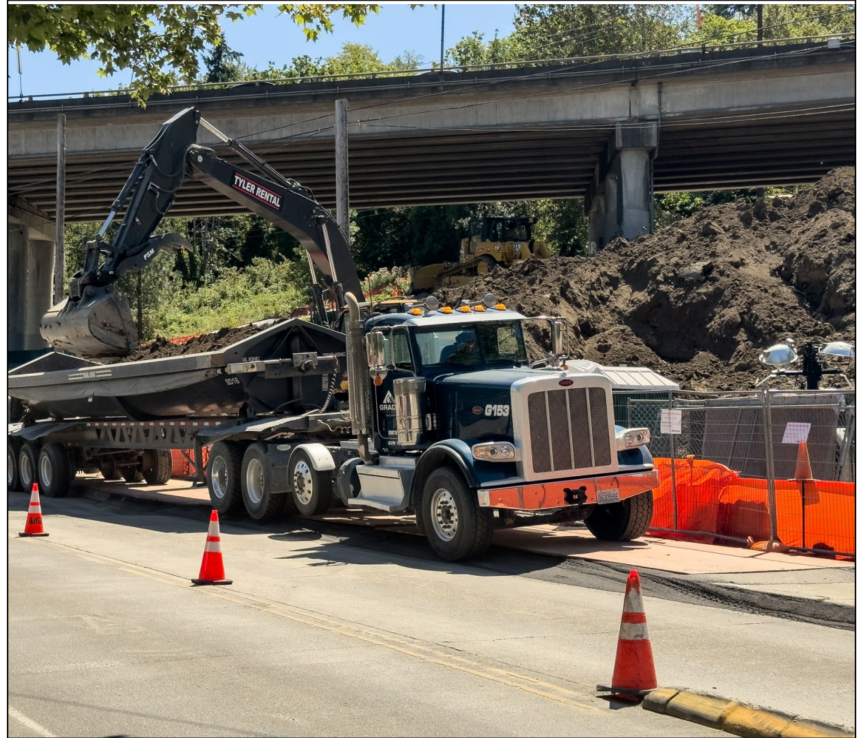
Excavation work area near Boyer Avenue East, looking southwest (July 2026)
