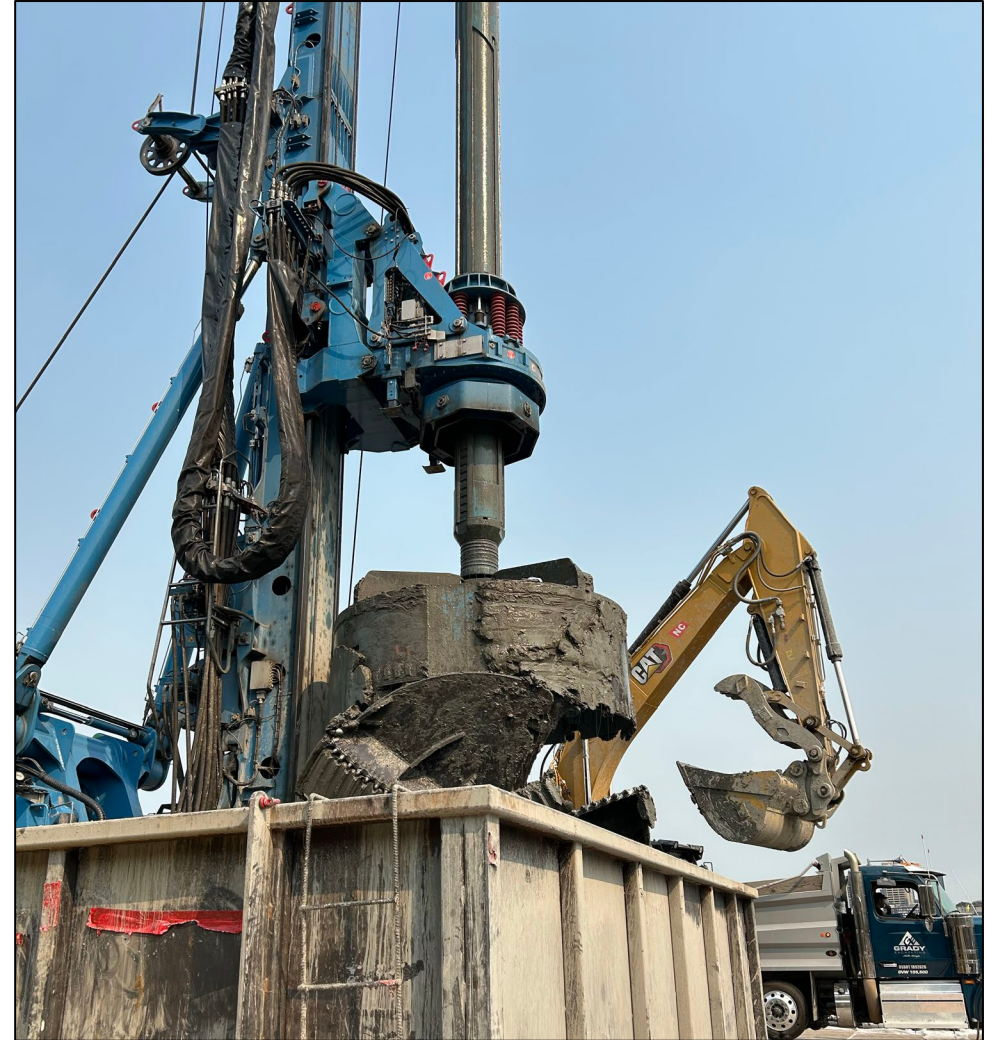
Crews using a bucket grabber to remove soil from a drilled shaft casing (August 2026)
