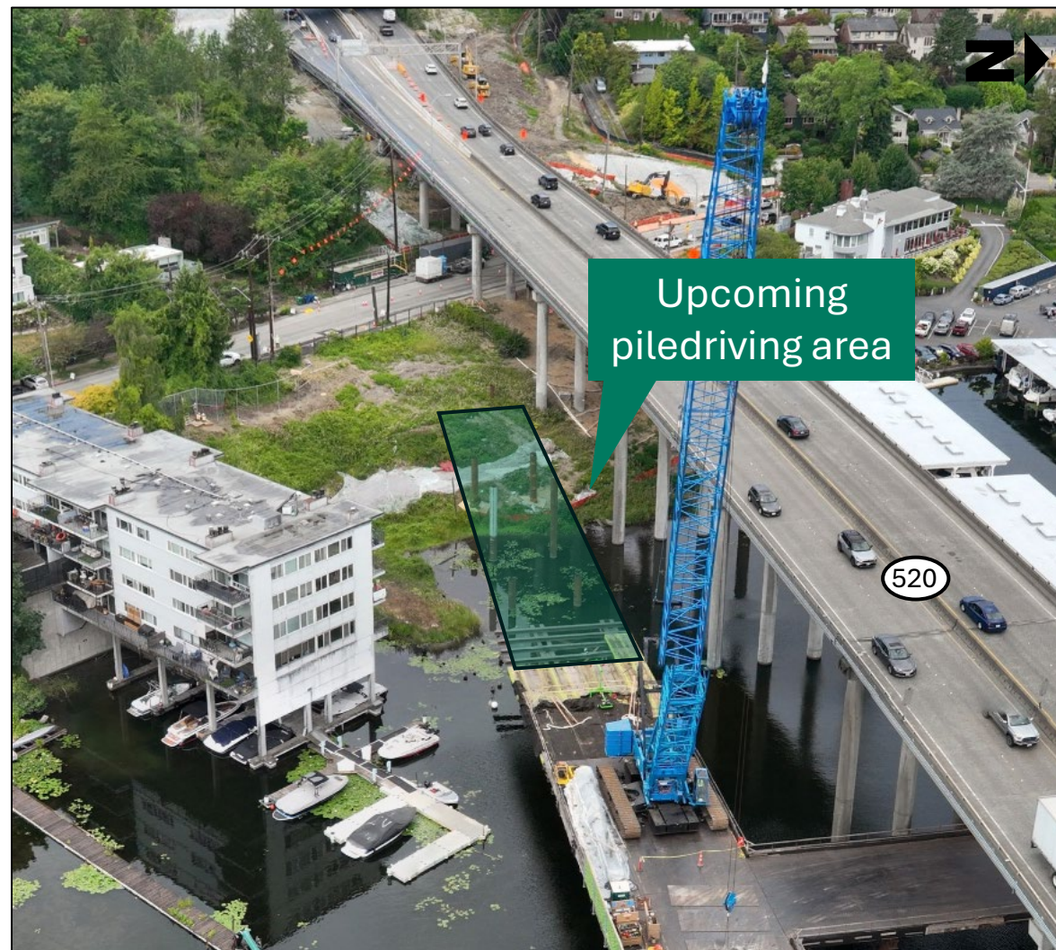
Graphic showing the piledriving area between the work trestle and Boyer Avenue East.
