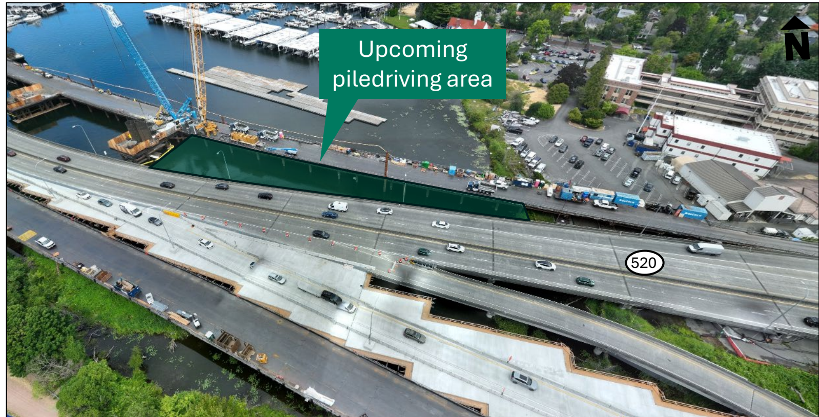
Piledriving area along the work trestle near the Montlake Lid.
