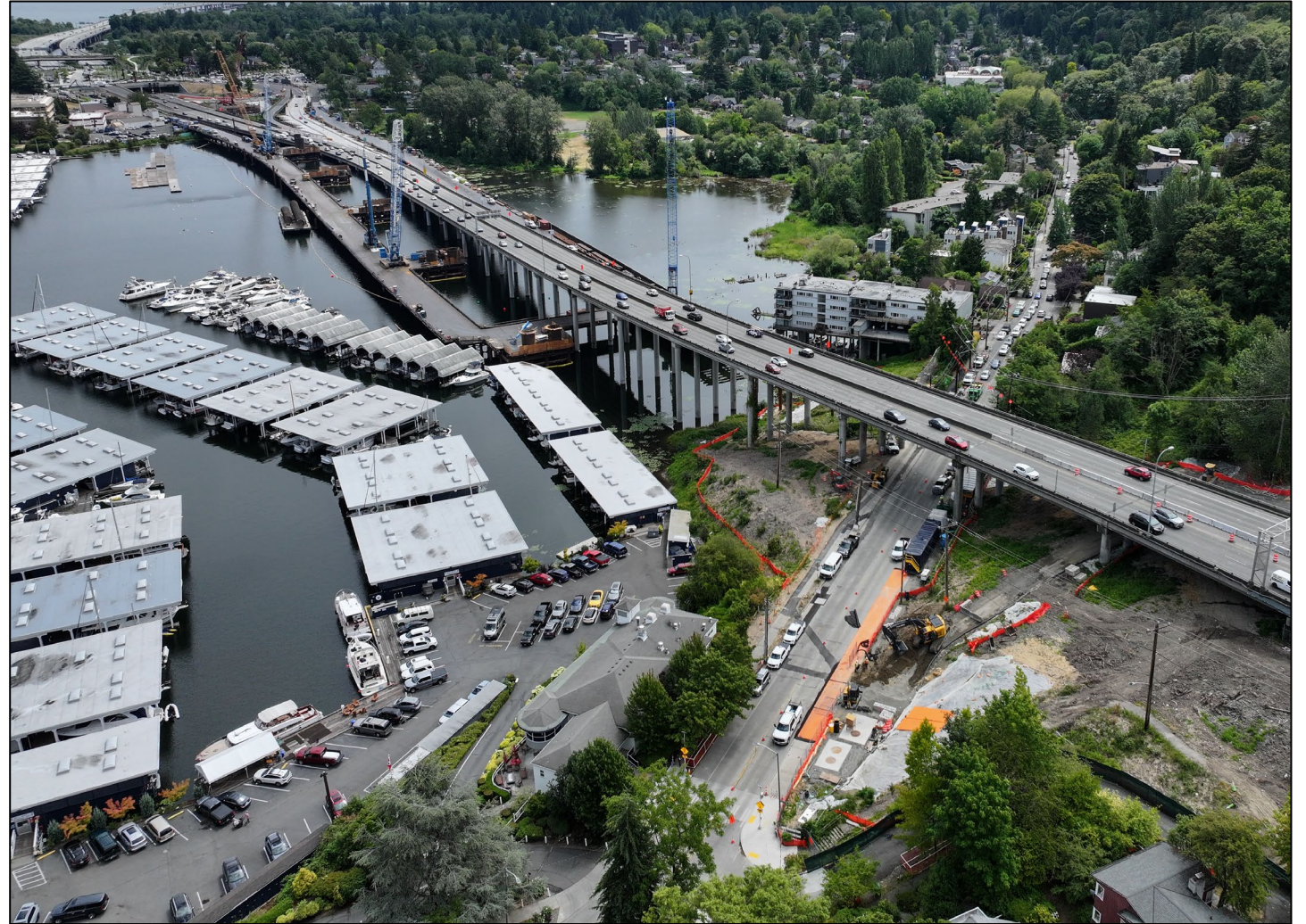
The Portage Bay Bridge project area looking southeast (July 2026)
