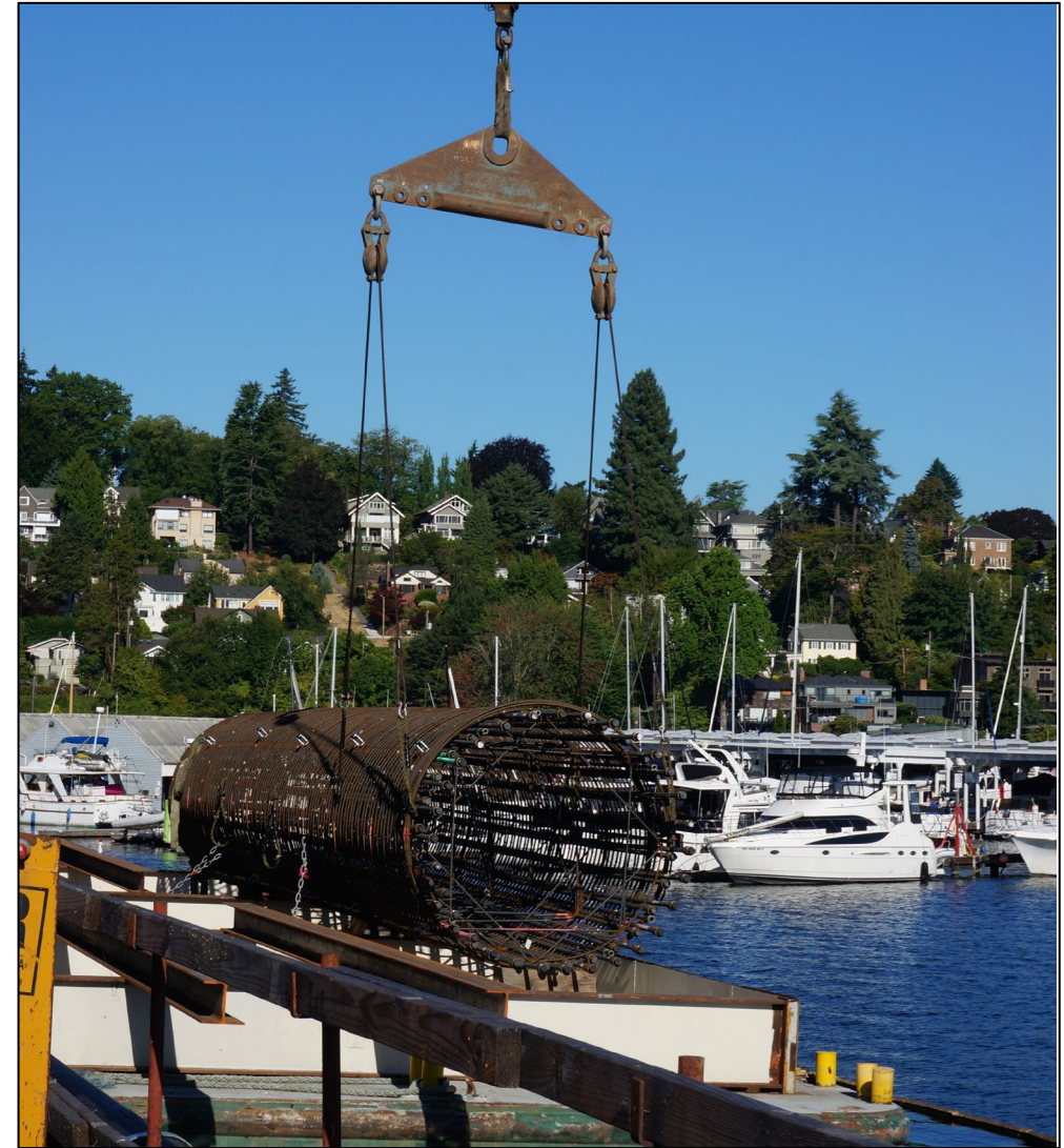
Crews using a crane to move a rebar cage to the work trestle (June 2026)
