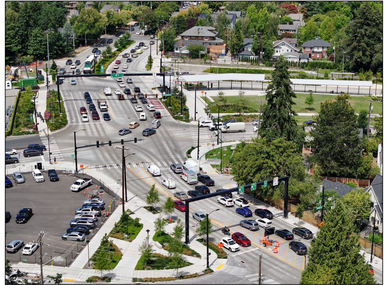
Aerial view (looking north) of Montlake Boulevard
