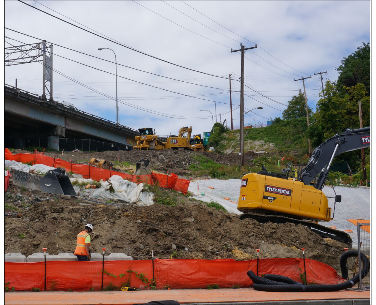
Crews working on the Boyer hillside (July 2026)
