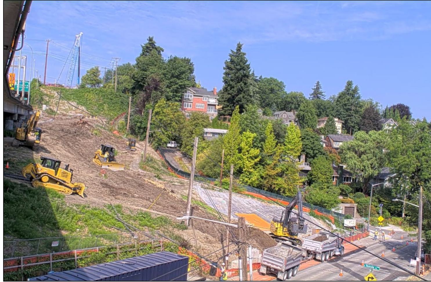
Excavation work area near Boyer Avenue East, looking northwest (July 2026)
