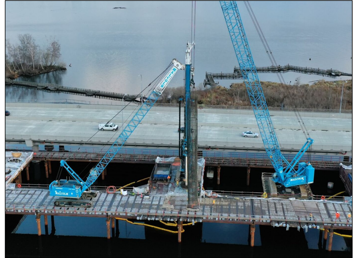
An example of crews using cranes to install rebar cages into casings (Source: Malcolm)
