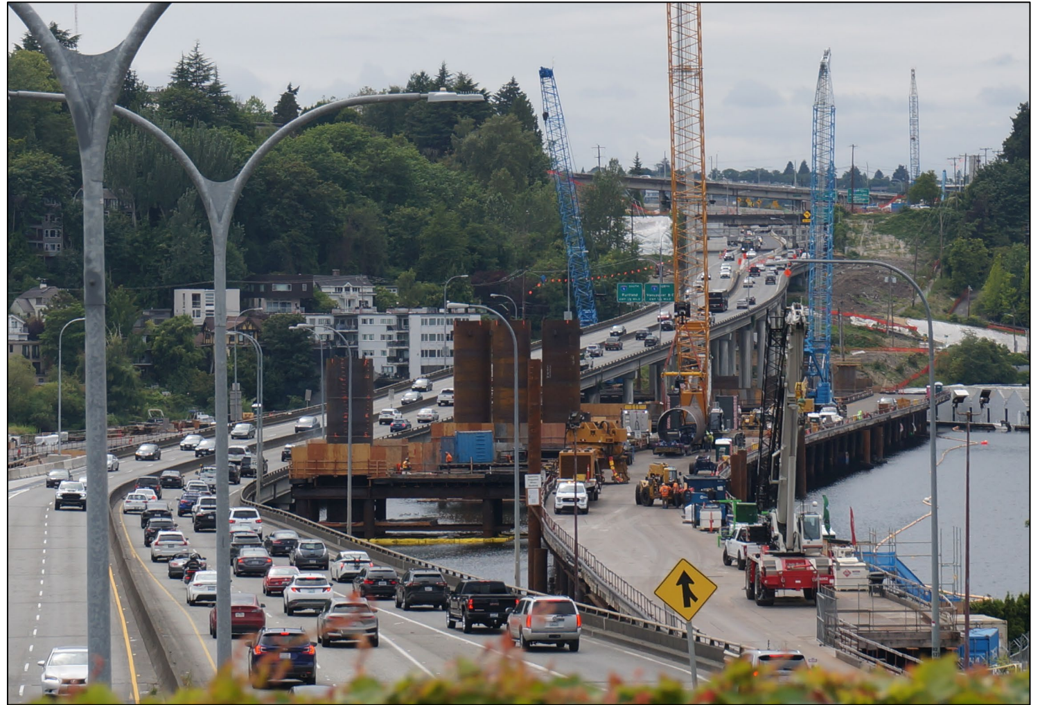
Three casings staged and cranes on the work bridge (July 2026)
