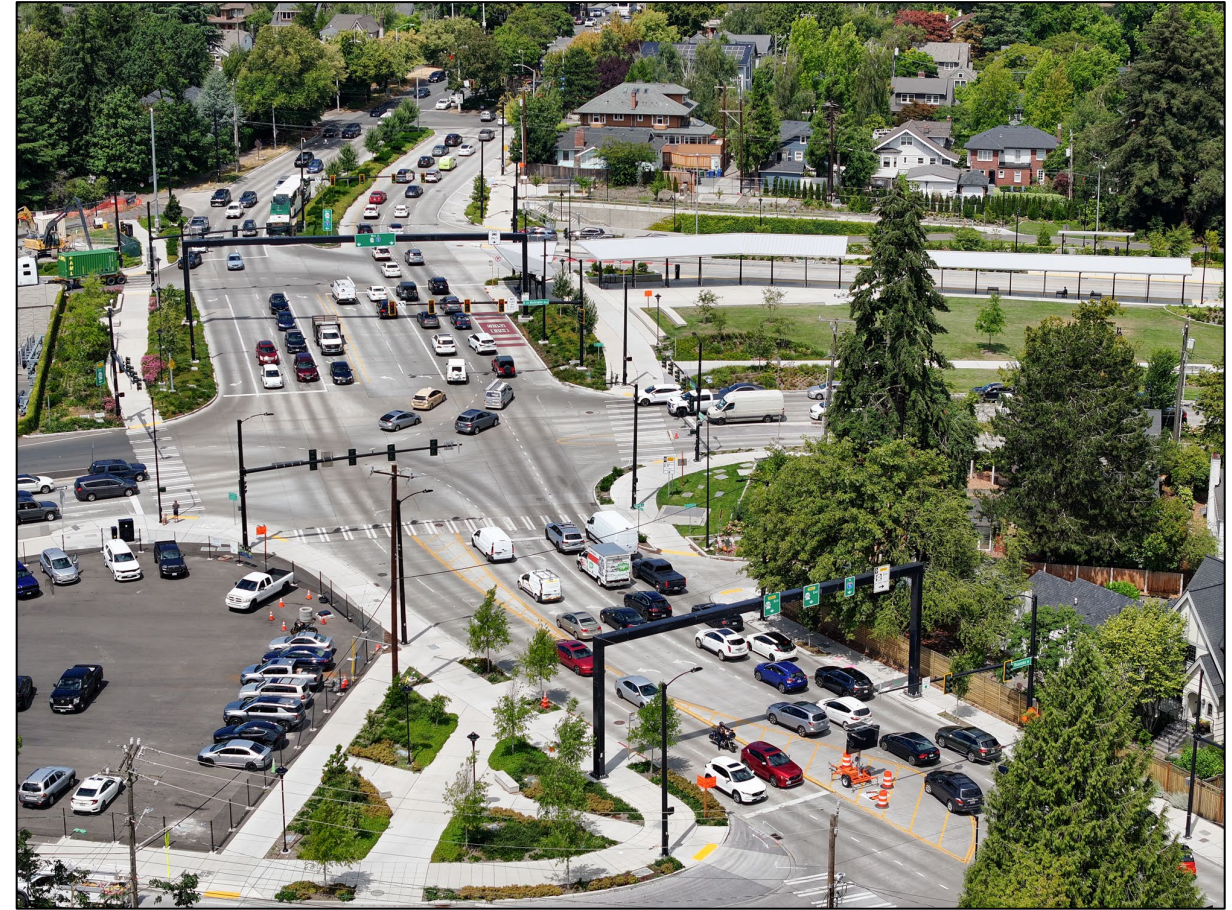
Aerial view (looking north) of Montlake Boulevard
