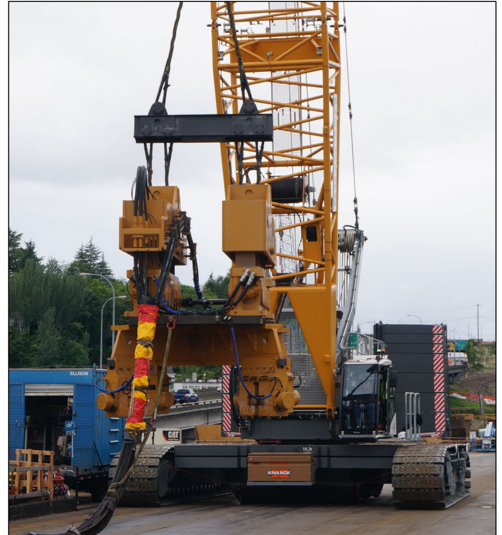
Crews using a crane to move the vibratory hammer between casings (June 2026)
