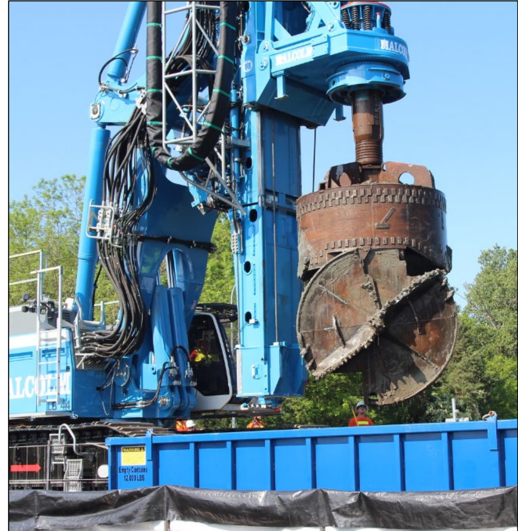
An example of crews using a bucket grabber to remove soil from a drilled shaft casing (Source: Malcolm)
