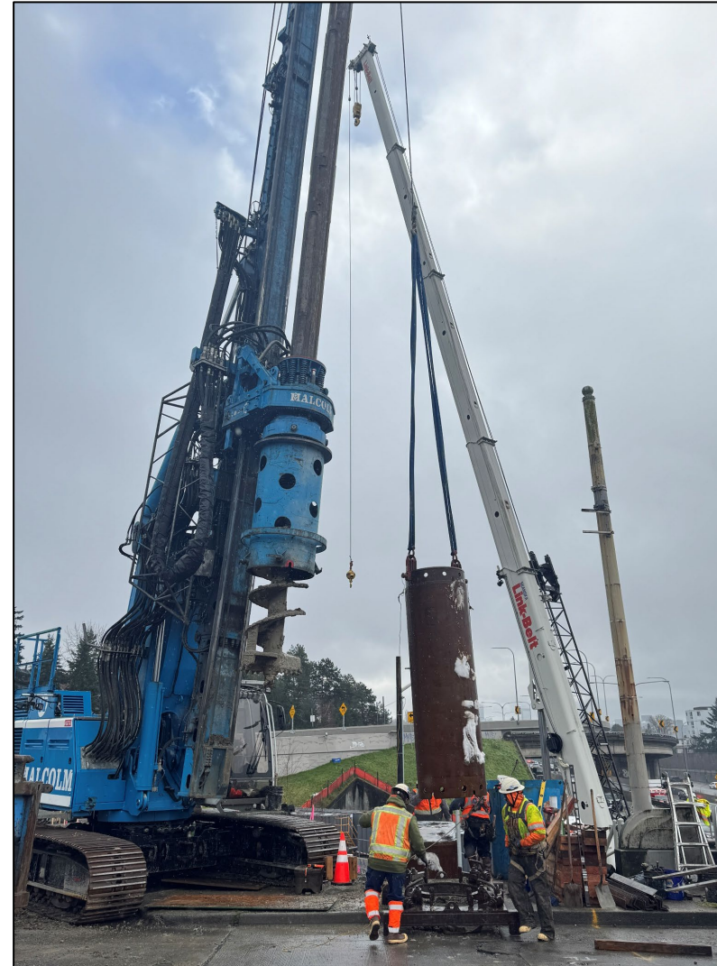
An example of the drilling equipment crews will use to construct the lid foundation (March 2025)
