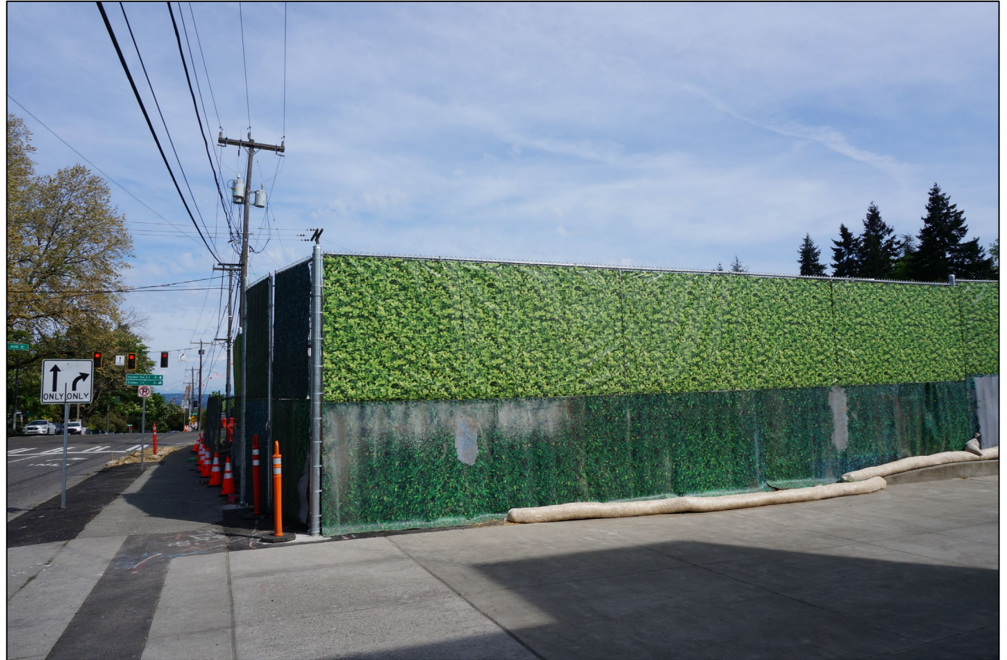
Acoustifence installed along E Roanoke St. (May 2026)
