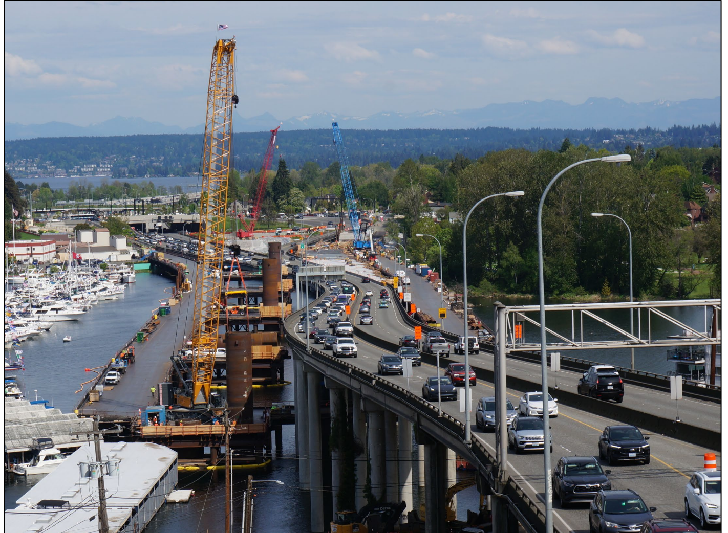
Crews install drilled shaft casings north of the Portage Bay Bridge (May 2026)
