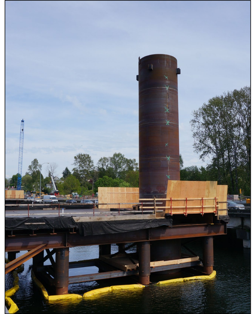
A section of casing prepared for vibratory hammer installation (May 2026)
