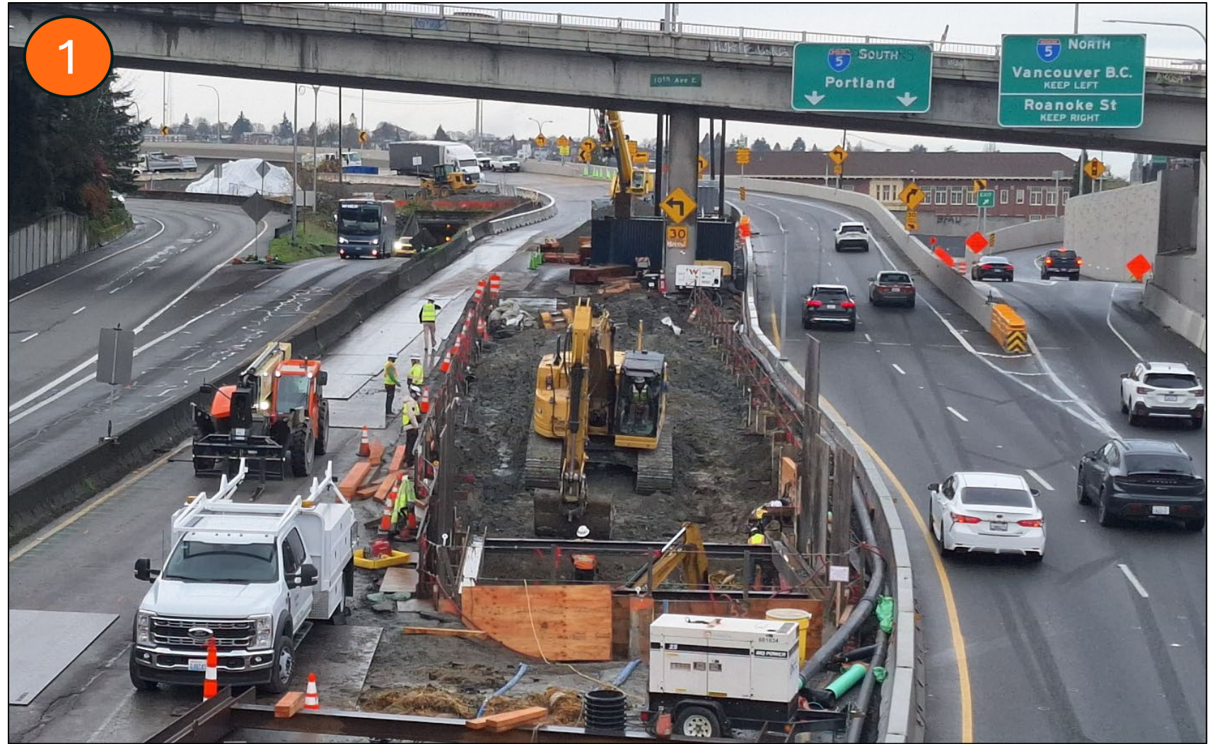
Crews excavating for the lid foundation between the eastbound and westbound lanes of SR 520 (Dec. 2025)
