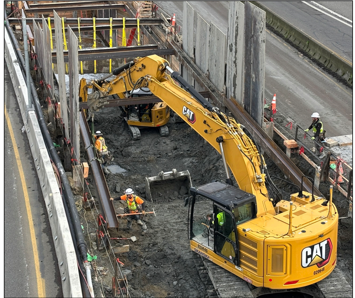
Crews excavating for the lid foundation between the east and westbound lanes of SR 520 (Jan. 2026)
