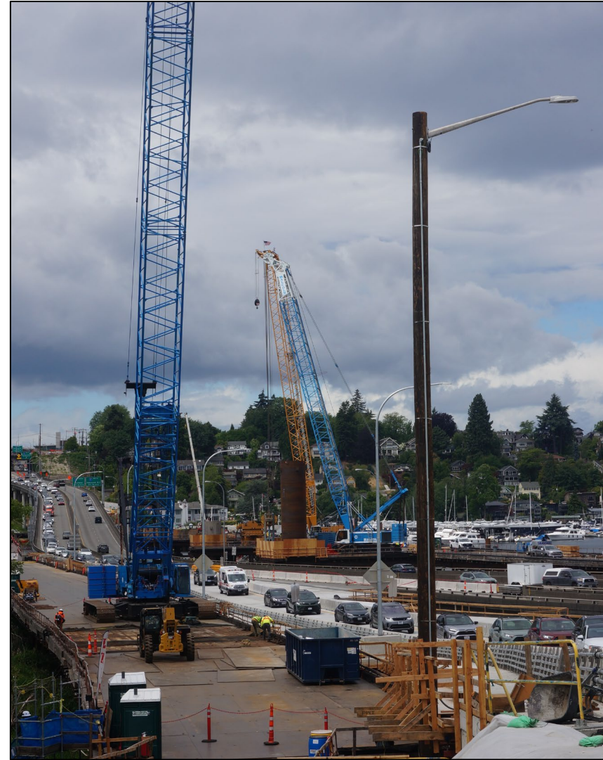
Crews using cranes to install casing sections (June 2026)
