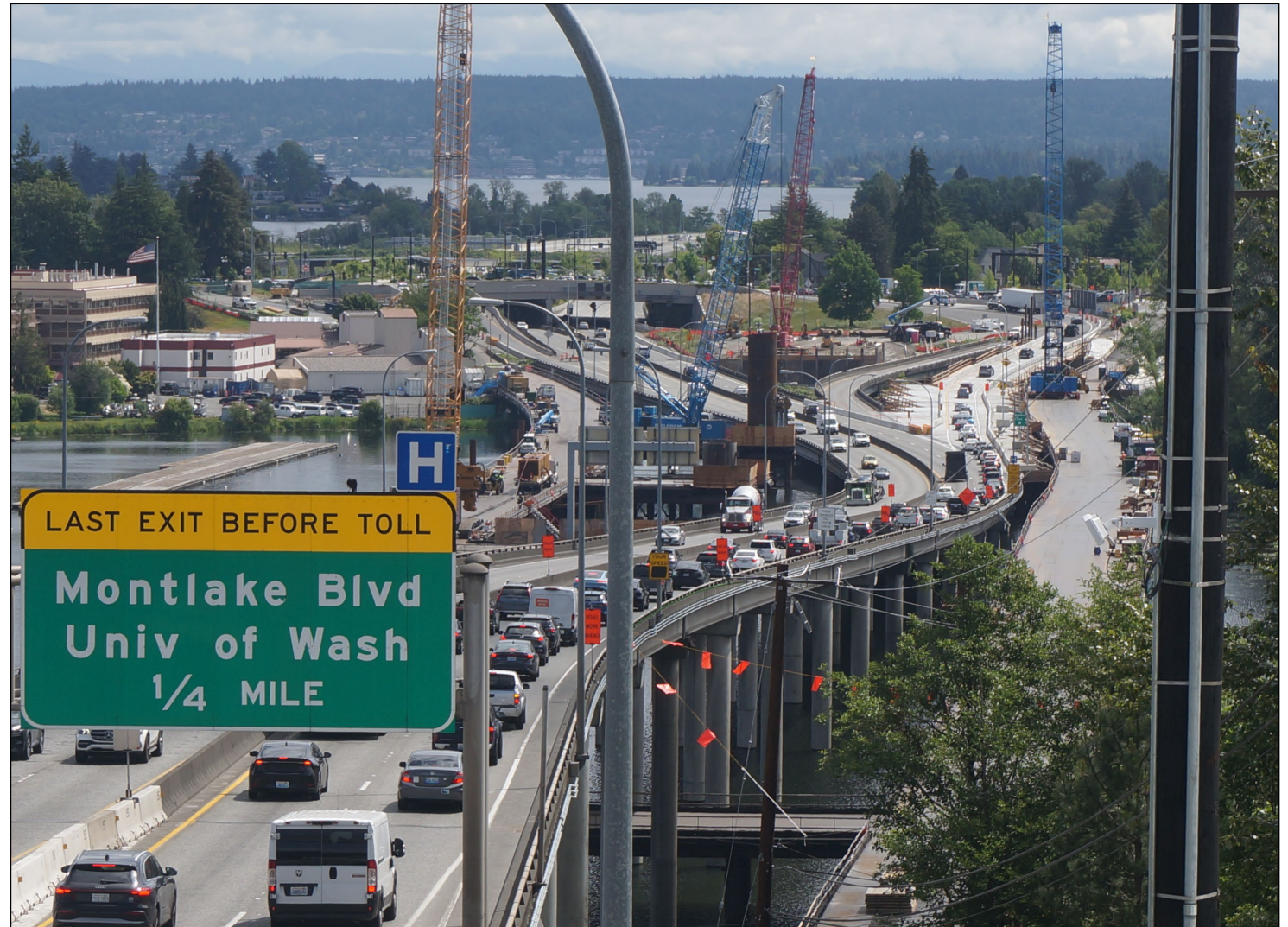
The new temporary off-ramp and existing bridge looking east (June 2026)
