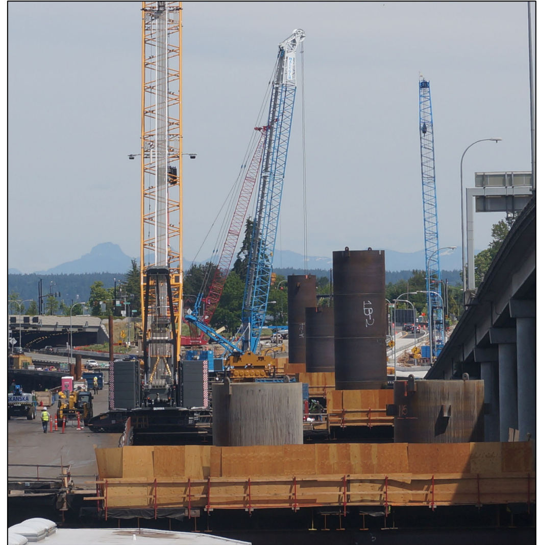
Crews installing casings (June 2026)
