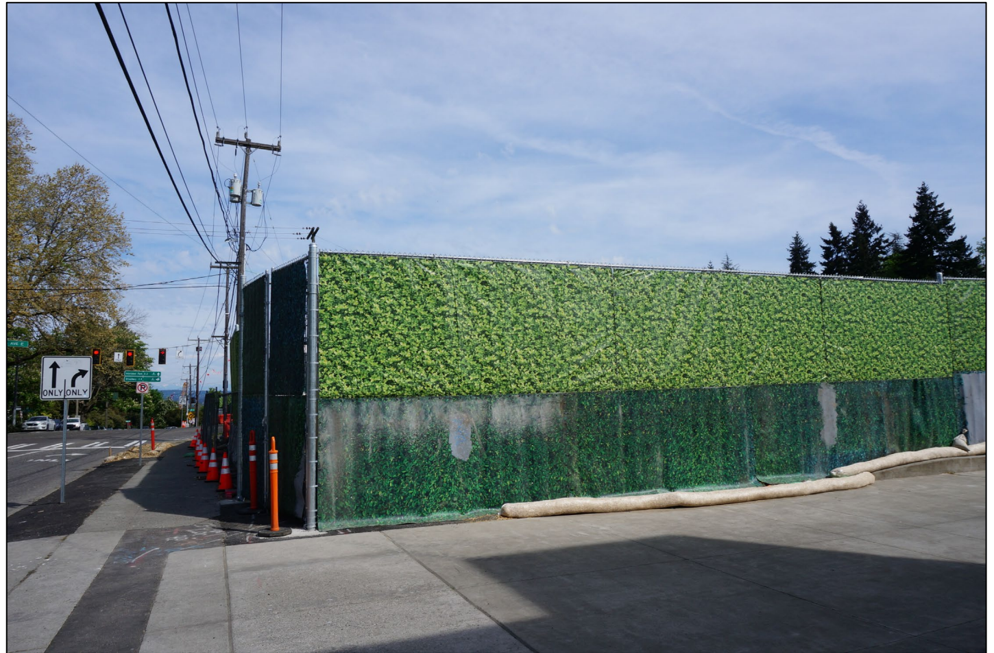
Acoustifence installed along E Roanoke St. (May 2026)
