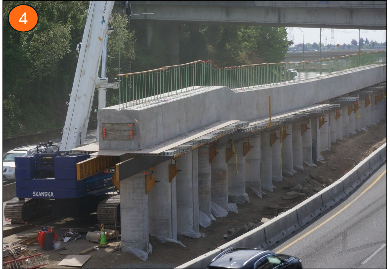
The foundation section with removed pillar forms, plates and beams (April 2026)
