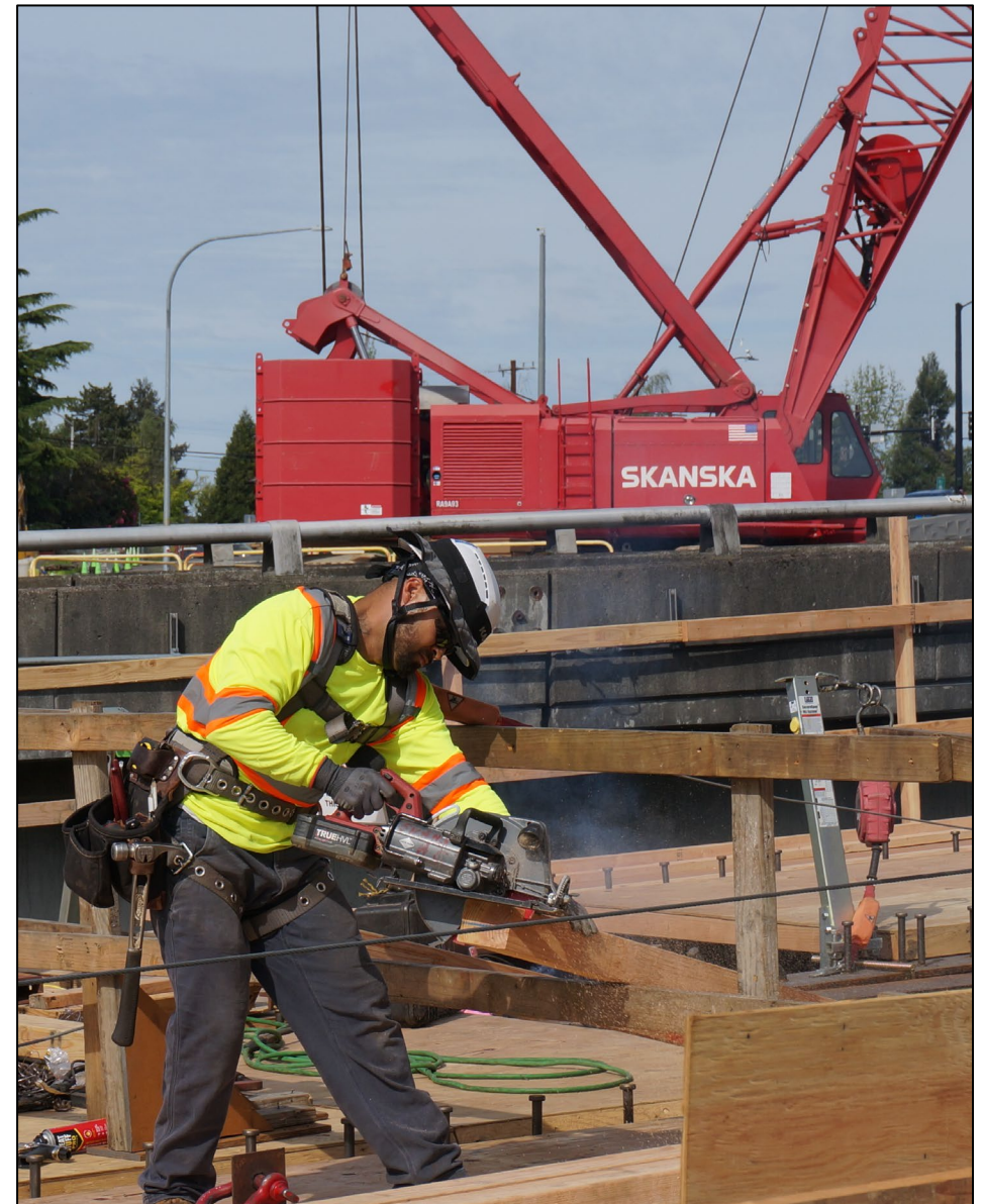
A worker builds framing for the new temporary SR 520 off-ramp (May 2026)
