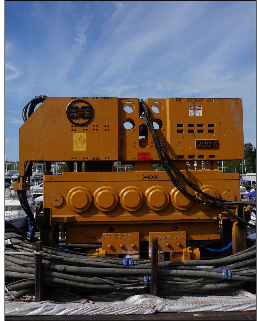
The vibratory hammer used to install sections of casing (May 2026)
