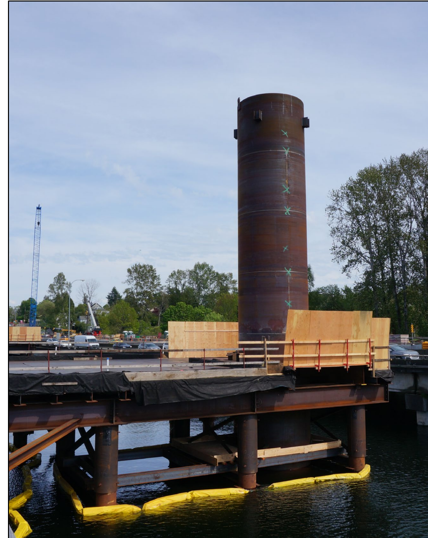
A section of casing prepared for vibratory hammer installation (May 2026)
