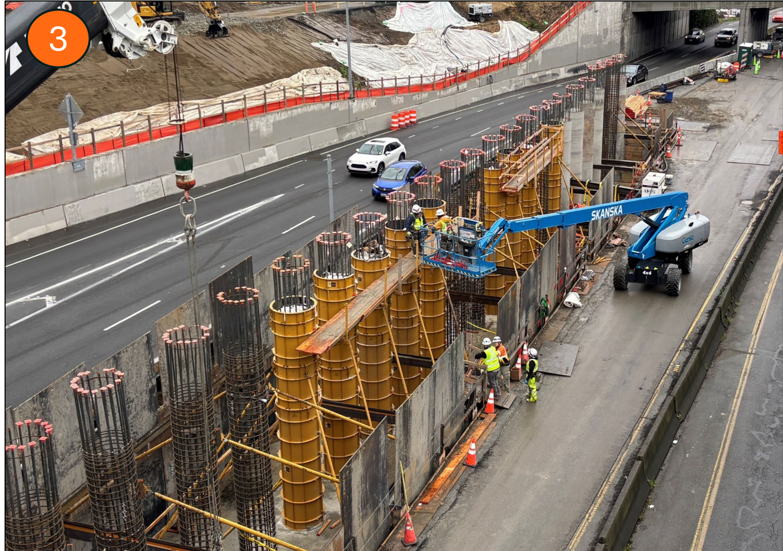
Crews placing pillar forms for poured concrete (March 2026)
